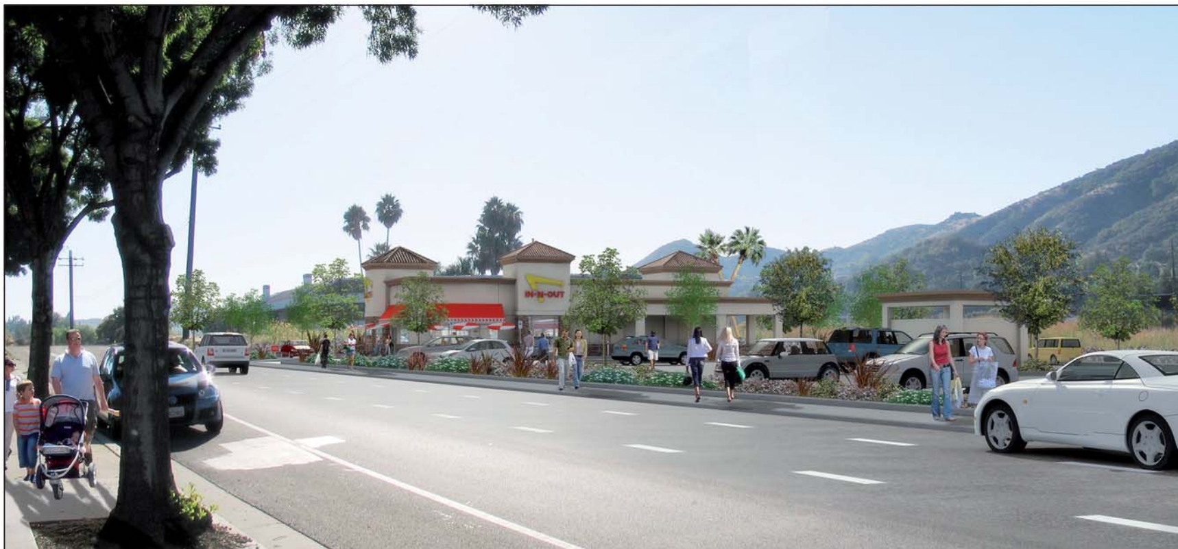
View of project looking east from Canwood Street.
